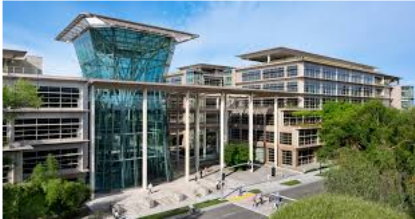
Photo from online images: CALPERS BUILDING, SACRAMENTO
